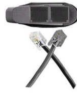
Wrong Wiring but Functional
